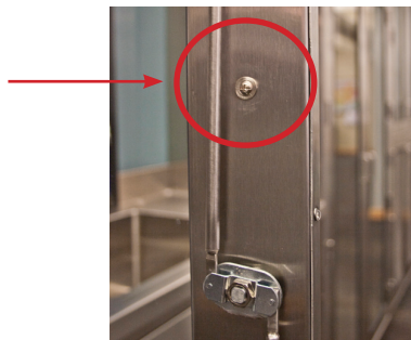
Fig. 27: Upper Fixing Bolt
